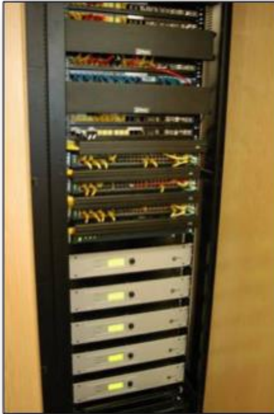
MPR – Central Rack per floor for Ethernet Switches and Mix Engines
