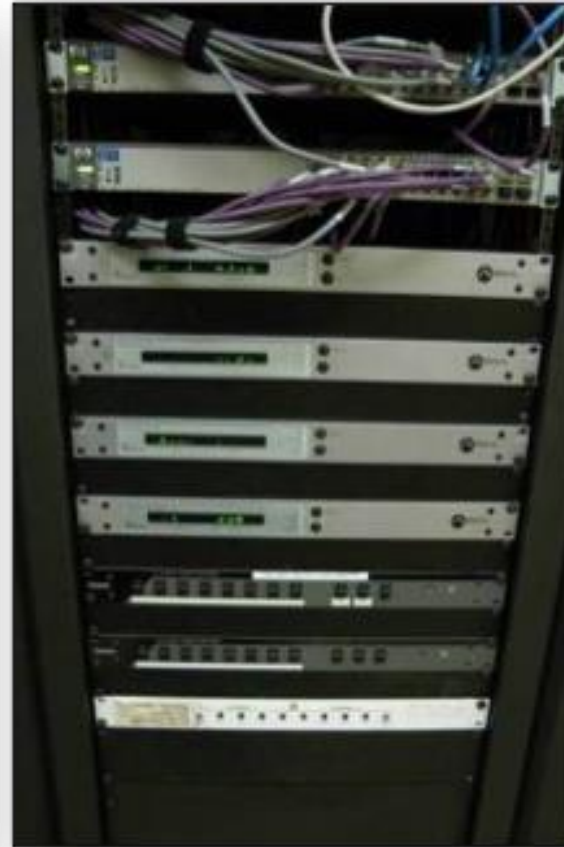
WICR-FM, Indianapolis Rack with Ethernet switches and Tech Center nodes.
